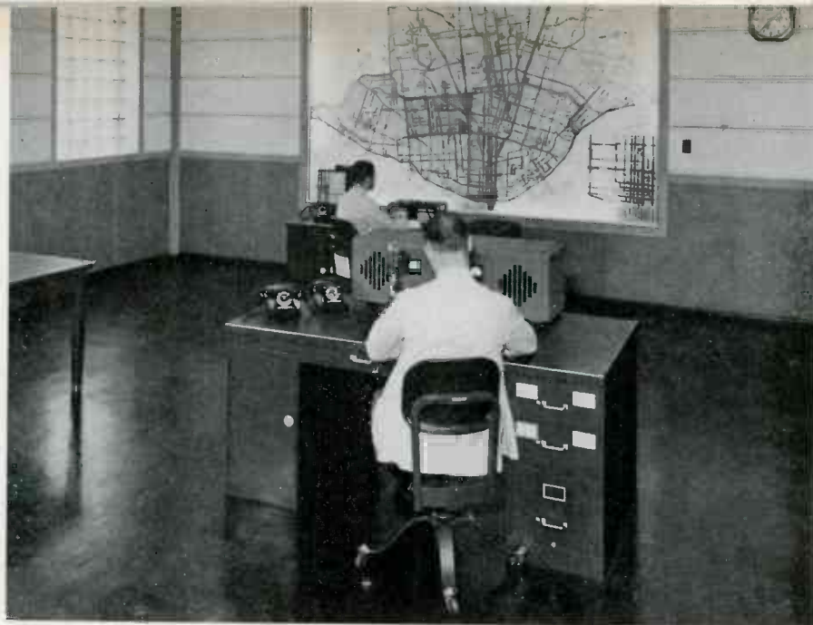
The main transmitter (left) for the St. Louis Public Service Co. Radio Station. This unit, which is unattended, is remotely controlled by the console in the dispatcher's quarters (shown above). The illuminated map shows the entire street car and bus system of the company. It is divided into ten districts by means of different colors, each district being under the supervision of one of the radio cars.
